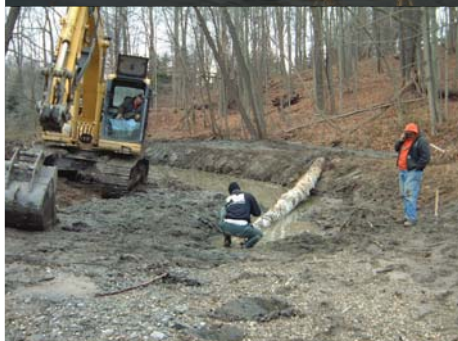
Silver Creek during construction
