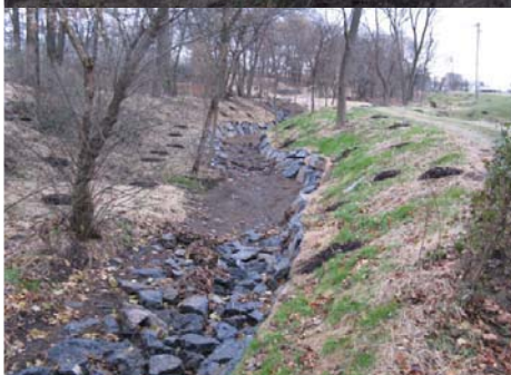
Valley Road stream channel after restoration
