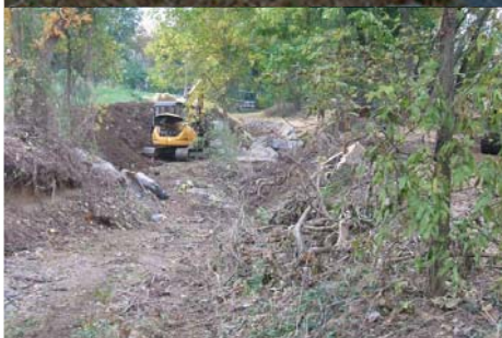
Valley Road stream channel during construction, a Biohabitats/Meaville design-build
