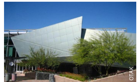
Tempe Transit Center
